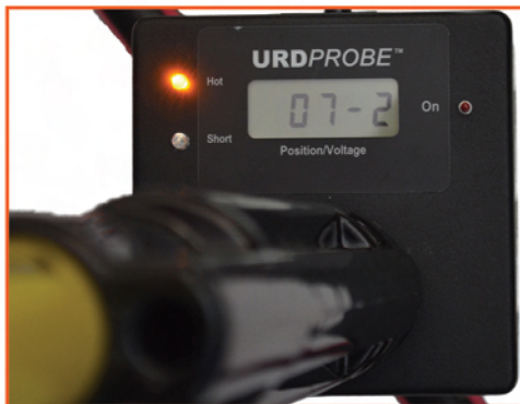
Indicates approximate voltage as 7.2KV.
