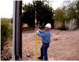
An APS electric troubleman dedicated to the remote phase ID project prepares to acquire phase information and GPS location of the measurement.
