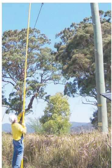
Using the PhaseID System to identify the phase of a feeder wire.
